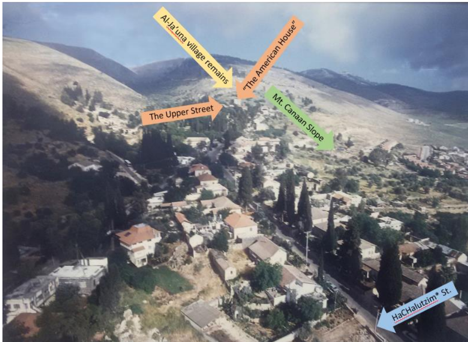
Illustration 3: Rosh Pinna – view to the west (photograph courtesy of the Rosh-PinnaRosh Pinna Local Council)
